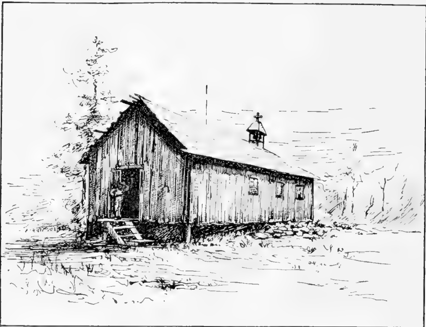
FIG. 68.—Shaker church at Mud bay.
